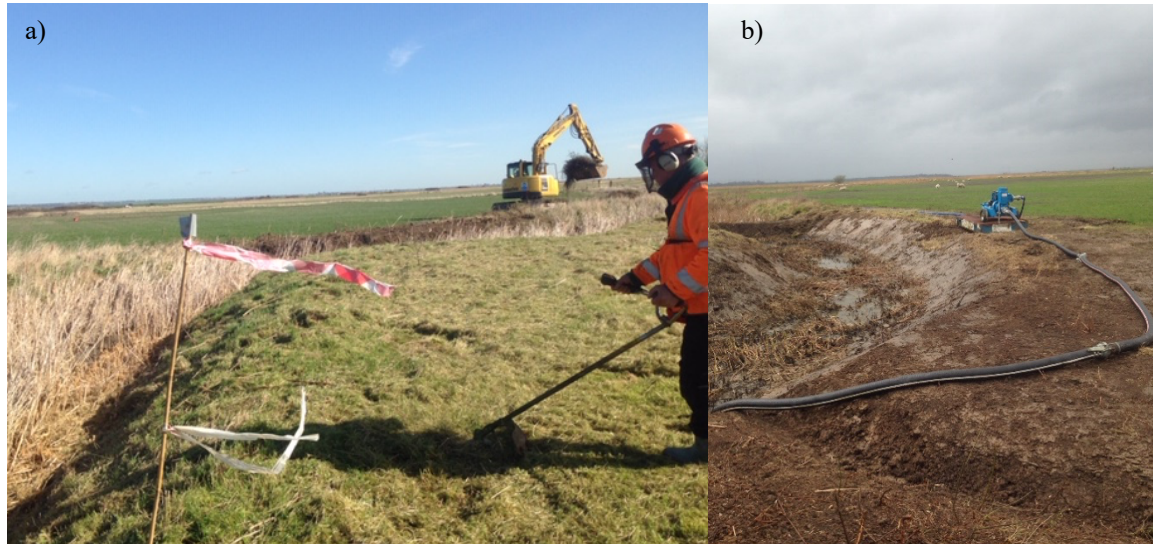
Figure 1: Displacement Area, a) prior to surface scrape and water drawn down, and b) subject to surface scrape and removal of water. Photographs: Charlie Dwight
