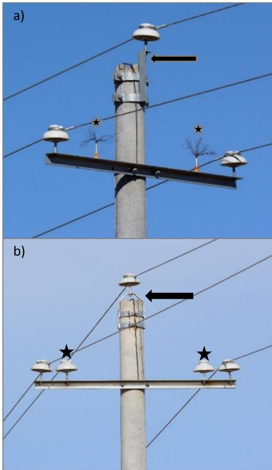
**Figure 1.** a) Control line pole with side-mounted single pin insulator at the top of the pole (indicated by arrow), and single pin insulators with pre-existing 'insulated brush' perch deflectors (indicated by stars) on the crossarm. b) Mitigated line pole, with centrally mounted pin insulator (arrow) at the top of the pole and additional unconnected pin insulators (stars) on the crossarm.
