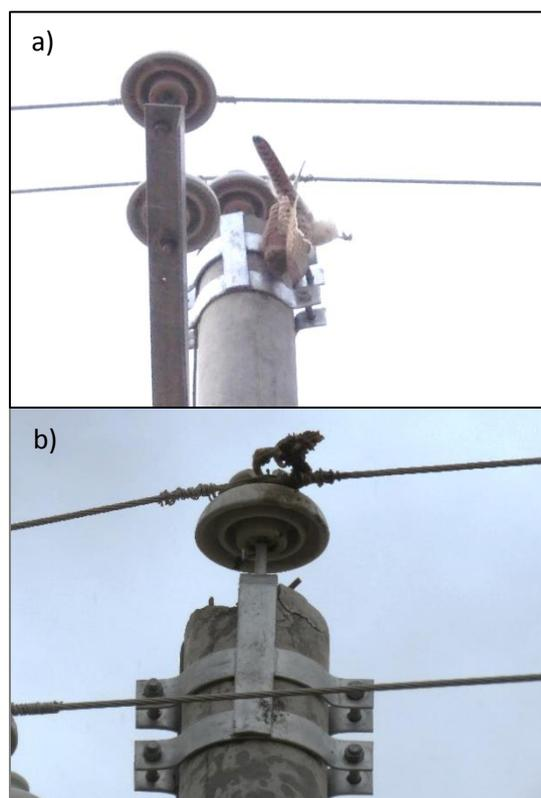
**Figure 2.** Evidence of raptors electrocuted at the top of mitigated poles: a) common kestrel electrocuted when perched on the bolt-bracket for the arch-shaped pin insulator mount. b) golden eagle talon still attached to phase cable after electrocution when perched on the pin insulator while carrying a large prey item (eagle carcass with steppe polecat prey found below pole).
