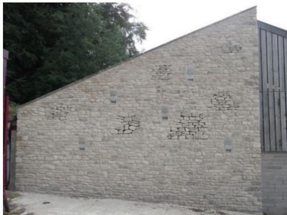
Figure 3. New purpose-designed Bat Wall constructed on the east-facing gable wall of an existing hay barn; includes multiple crevices between the stonework leading to internal cavities and five wall integrated IFR Schwegler Bat boxes.
