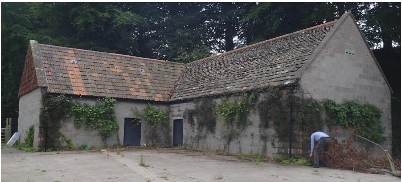
Figure 2. New purpose-designed 'L' shaped Bat House including a sloping gable roof (longest section is east-west aligned); visible roost features include bat tiles, ridge beam access points, wall-integrated 2FR Schwegler Bat boxes, hanging tiles, and wall mounted climber planting.
