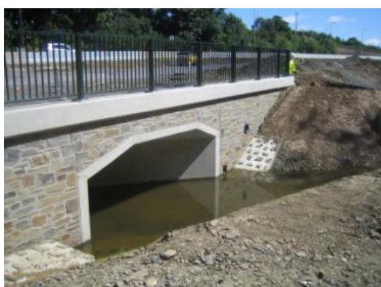
Figure 4. Toch Brook box culvert.
