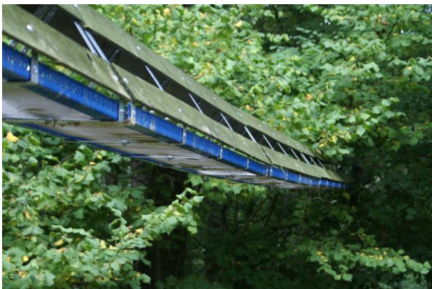
Figure 4. Photograph of end of trial dormouse bridge, well connected into surrounding dormouse habitat network.
