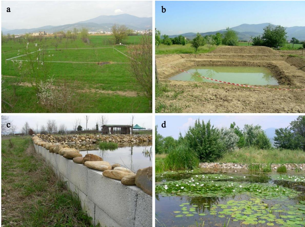
**Figure 1.** Site 1; a) before the intervention, b) the digging completed, c) detail of the barrier, d) spring 2012, three years after the site was created.
