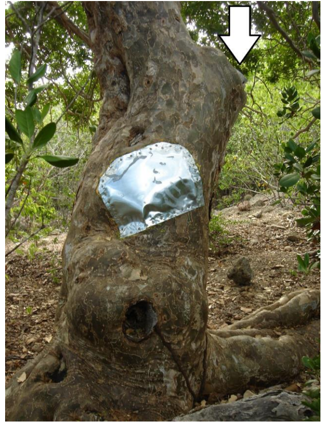
Figure 2. Repaired yellow-shouldered Amazon nest cavity, with metal sheet covering the hole. The metal sheet was then painted to make it blend in with surroundings. Arrow indicates nest entrance.
