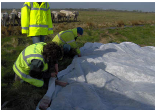
Figure 2. Bricks are attached to the bottom of a geotextile membrane to provide a weighted hem to a 'silt curtain', spring 2006.
