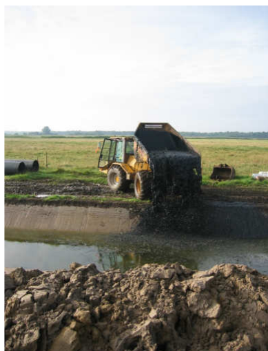
Figure 5. Silt from the old soke dyke (containing pondweed turions) placed into new dyke to act as inoculate, August 2006.
