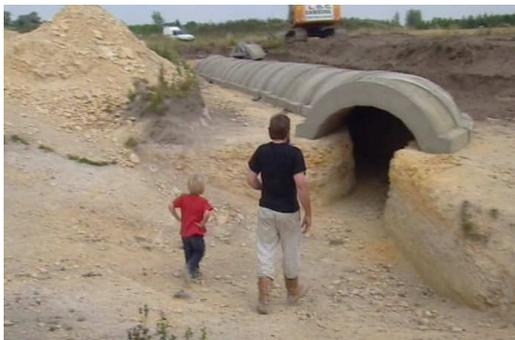
**Figure 1.** The hibernaculum was created by digging a trench out of limestone and by putting pre-cast concrete roof sections over the trench.
