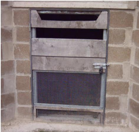
**Figure 3.** Cave door made of steel and oak boards. The top has two slots for the bats to enter and exit the cave. The bottom is made of wire mesh to enhance ventilation.
