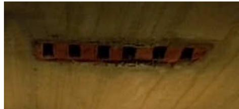
**Figure 2.** Bat brick, containing six gaps, each gap has room for 2 - 3 bats to hibernate within.
