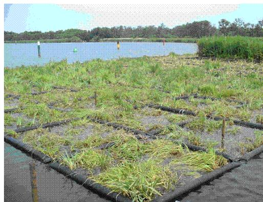
**Figure 1.** The floating island showing the plastic floats supported by metal grids and recently planted vegetation.
