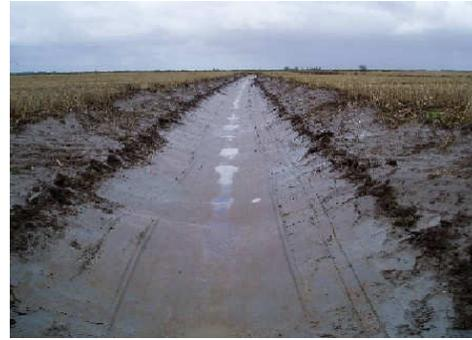
**Figure 1.** A recently excavated footdrain approx. 40 cm deep and cut using a rotary ditcher.
