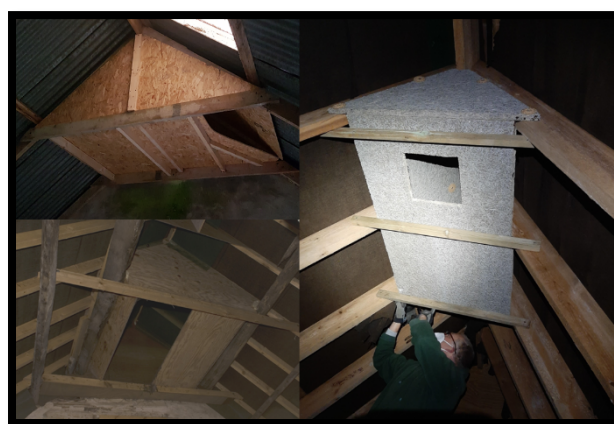
Figure 3. 'Hot boxes' of various design, installed into the apex of the roof interior at horseshoe bat roosts.
