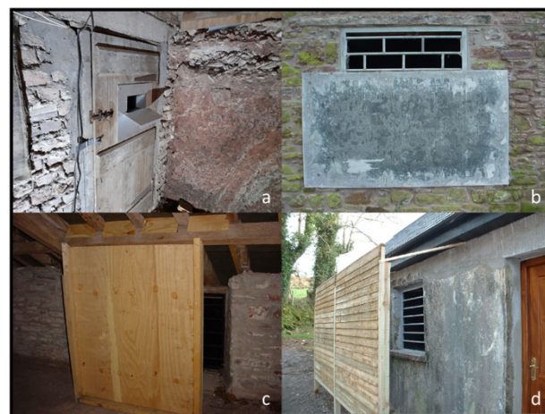
Figure 2. Entrance modifications to improve horseshoe bat roosts. Entrances can be made predator-proof by installing a 'tip tray' (a) and anti-climb surfaces (b). Grills can be installed to deter vandalism (b, d). Baffles can be installed to reduce draughts and light into the building (c, d).
