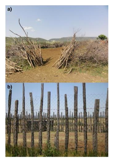
**Figure 2.** Contrasting Maasai boma styles: a) a traditional unfortified Maasai boma; b) a boma fortified in the Mara North by the Anne K. Taylor Fund using posts, chain link wire, galvanized wire, and immature thorny plants.
