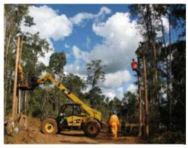
Figure 3. Construction of mine area lemur bridge.
